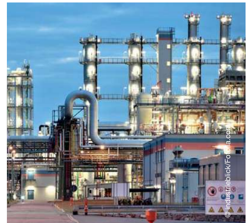
Compact and clever for the chemical industry: circuit breaker type 1180
